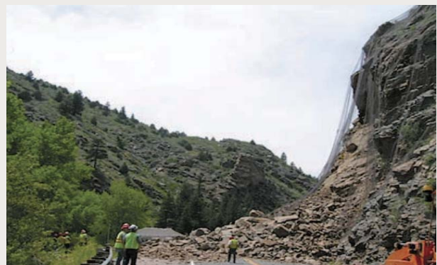
A rockfall that occurred in Clear Creek Canyon, Colorado, USA 2005
