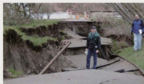
Example of lateral spreading, a type of ground failure often associated with earthquakes
