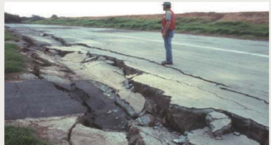
Lateral spread in 1989 in Loma Prieta, California, USA (Steve Ellen, U.S. Geological Survey)
