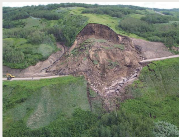
A translational landslide in 2001 in British Columbia, Canada
