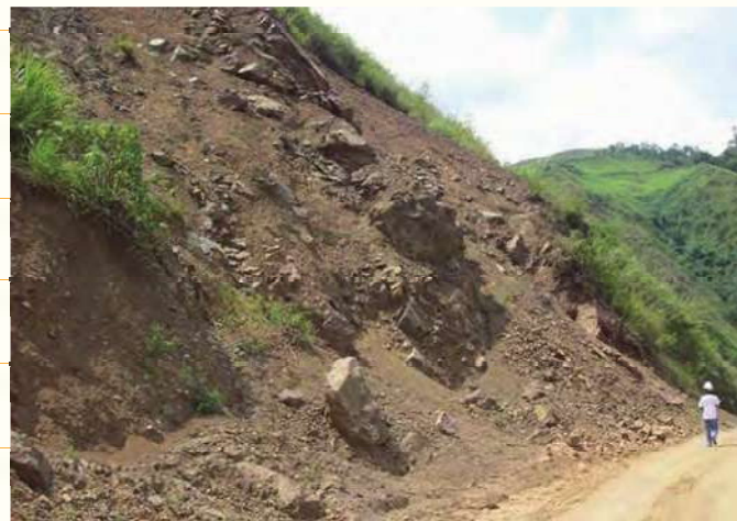
Figure 9-2: Samples of disintegrated, unstable and protruding rocks [source: DRH 61]
