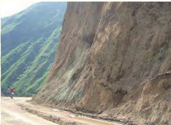
Figure 12-2: Sample photos of stiff, cemented and dense gravelly, sandy, silty and clayey soils [source: DRH 61]
