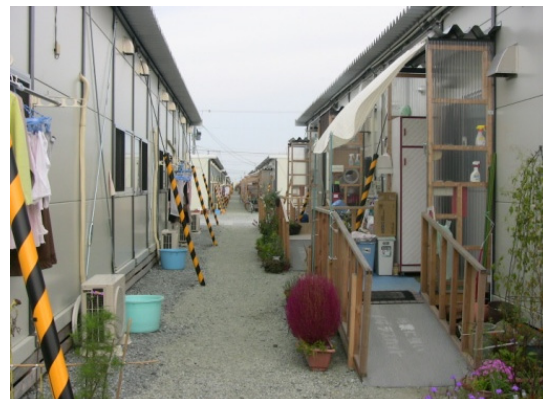
亶理町応急仮設住宅 Watari Temporary Housing
