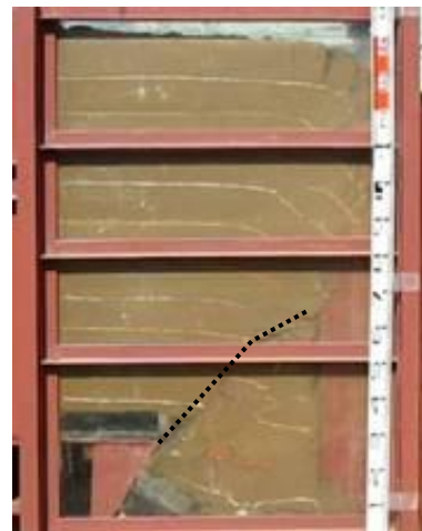
Photo 2 Fault part side
