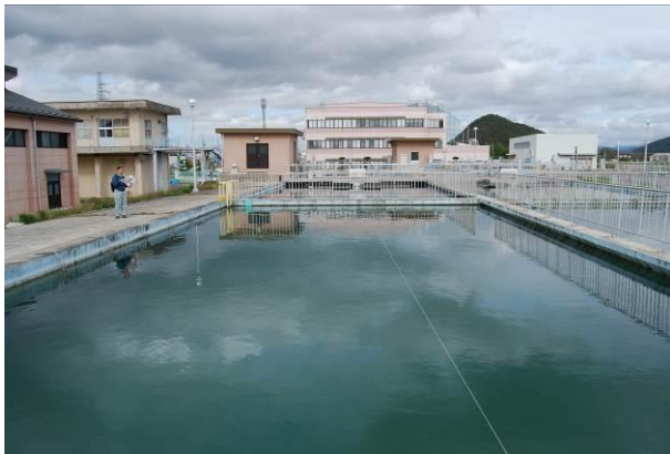
Photo 3 Sedimentation basin of the Hebita purification plant in Ishinomaki city
