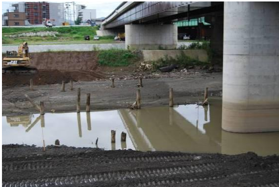
Photo 4 Former wood pile foundations near Kida Bridge
