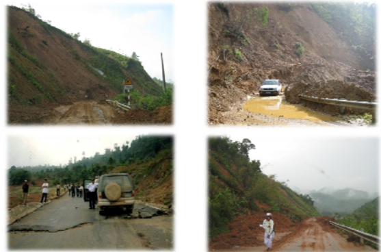
Landslide along Ho Chi Minh National Highway
