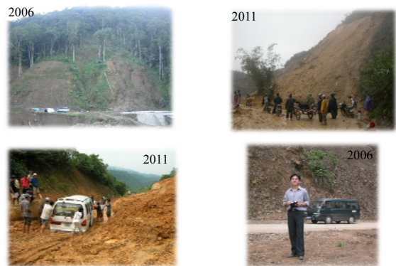
Landslide in Ho Chi Minh National Highway, Km399T+000
