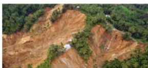
Landslide in Tandikat
