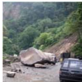
Rockfalls in roadway
