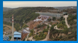
Yanlian landslide in Shaanxi Province triggered by water leaking
