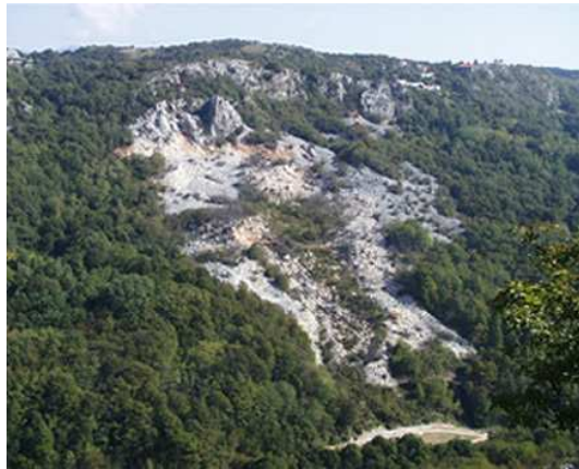
Figure 3.2 Photo of Grohovo landslide.
