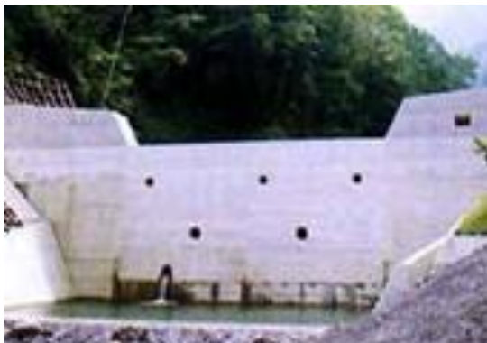
Fig. 3 Closed-type sabo dam
