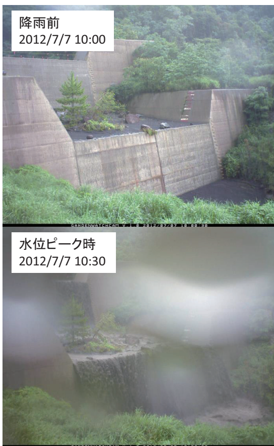
Fig. 7 Stream flow of Furusato River in July 7, 2012
