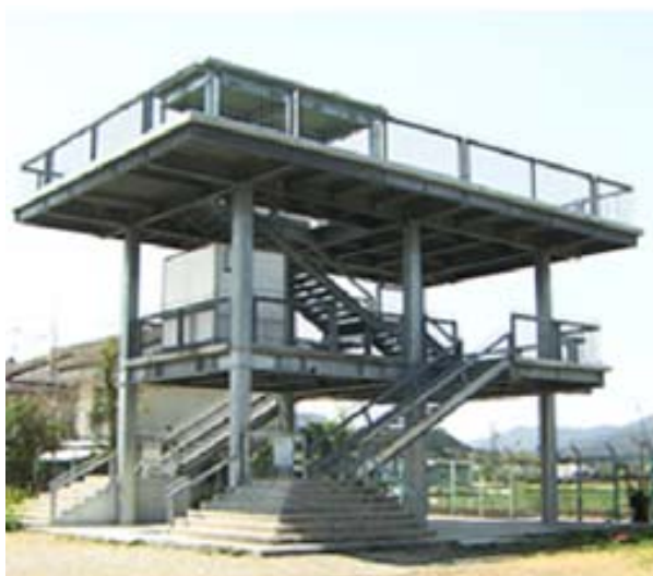
Fig 2. Current Tsunami Evacuation Tower
