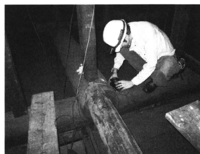
Photo1. Dr. Shimizu setting a precise velocity meter carefully on a roof girder.
