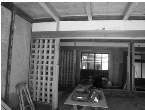
Fig.3 Inside view of the house under construction.
