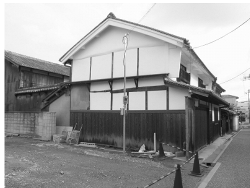
Fig.4 Outside view before renovation
