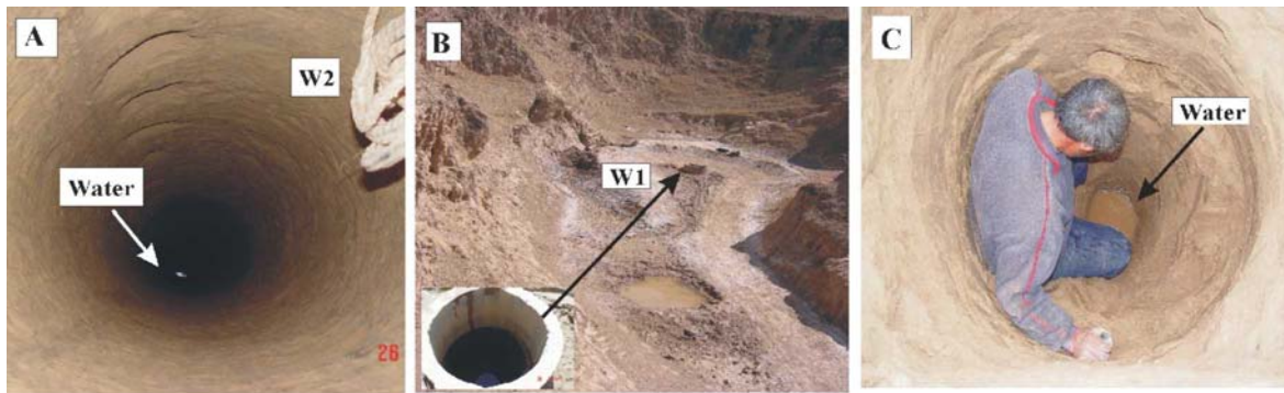
Fig. 5. Wells located in the right (a) and left (b) sliding blocks and the investigation pit (c) near the well W1
