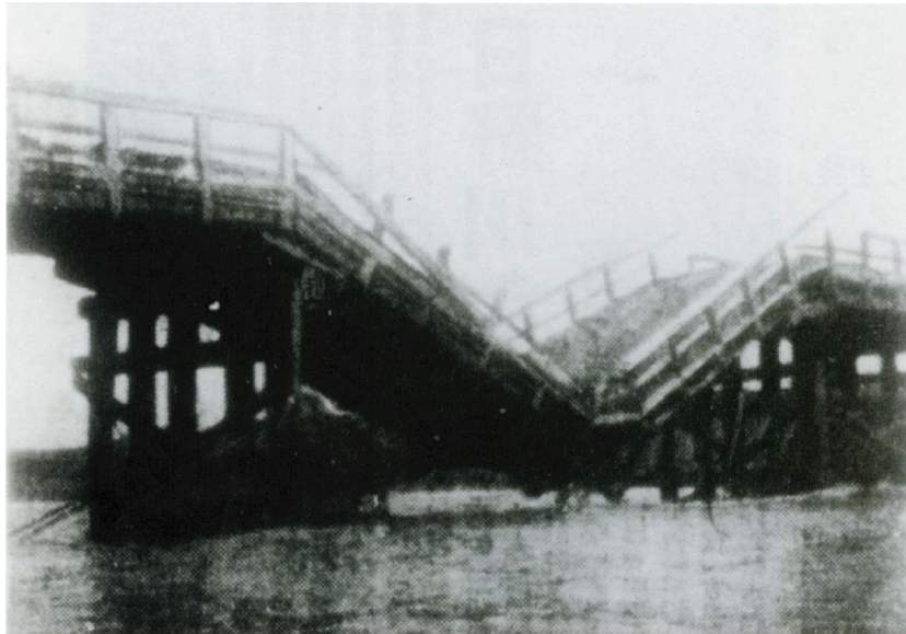
Picture 4.2 Ichimichi Bridge was damaged by Typhoon Isewan (1959)
