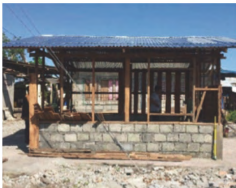
Figure 3 House under reconstruction by residents after Typhoon Yolanda
