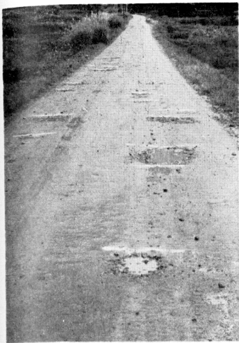
Photo. 1 Forest road R_1 before repairing road surfaces
