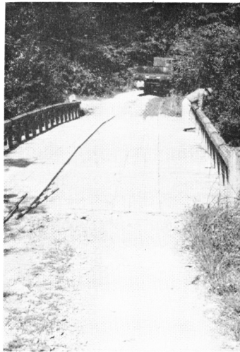
Photo. 9 Forest road, R_{11} , on wooden bridge
