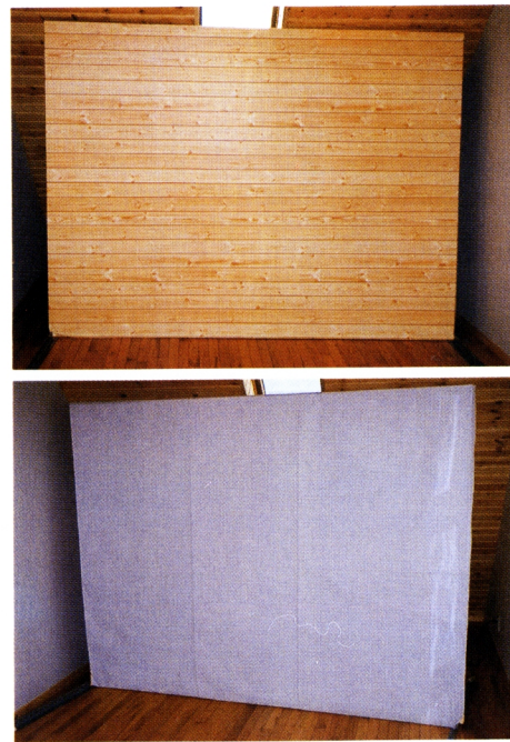
Fig. 4. パーティション (上:木目調, 下:和紙) Partitions. Upper photo: partition covered by wallpaper printed wood grain figure, Lower photo: partition covered by wallpaper made of Japanese paper.
