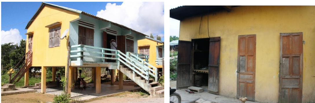
Figure 1.17. Provided house and auxiliary structure
