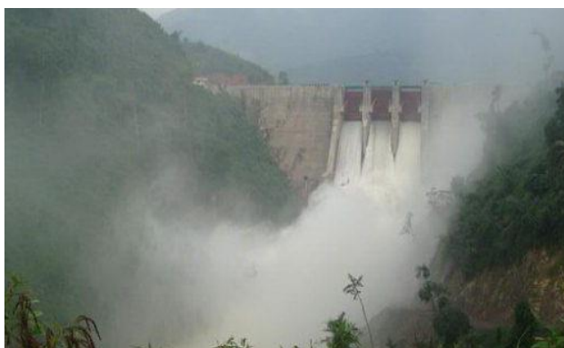
Figure 1.12. A Vuong dam release in September 2009 (Source: Viet Bao, 2009)
