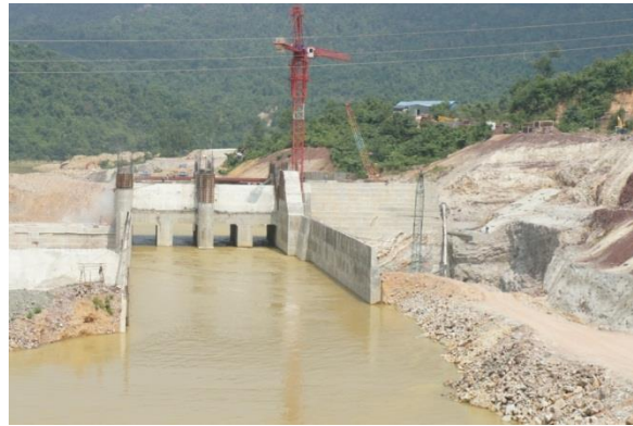
Figure 1.3. Dam under construction in Quang Nam province, central Vietnam
