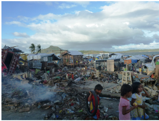
Photo 1 Damage situation in coastal area of Tacloban
