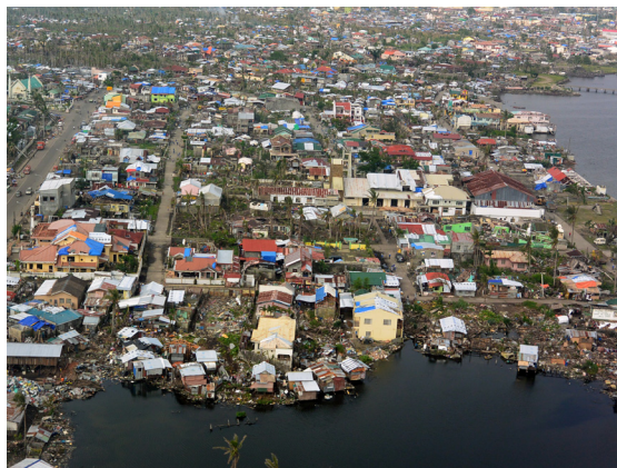
Photo 2 Aerial photo of coastal area of Tacloban
