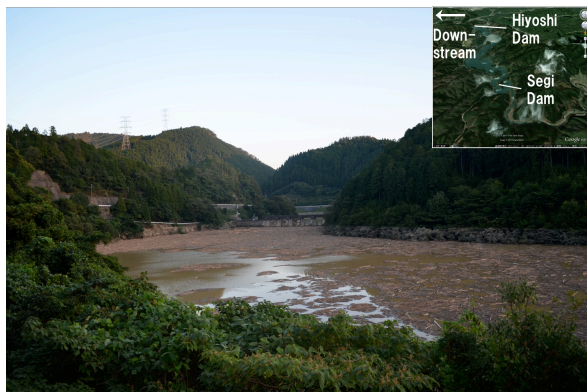
Photo 7 Accumulated driftwoods just downstream of Segi dam.
