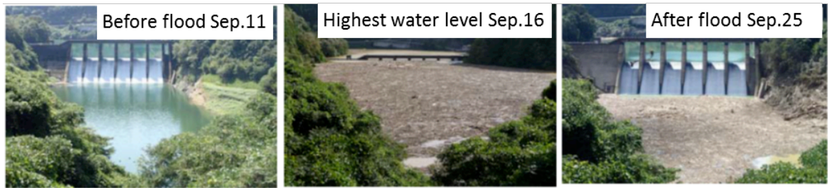
Photo 9 Accumulated drift woods in Hiyoshi dam reservoir just downstream of Segi dam (The Japan Water Agency).
