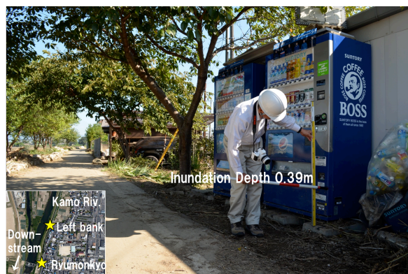
Photo 1 Inundation height on the left bank of the Kamo river near Shimo-Toba, Fushimi-ku, Kyoto city.
