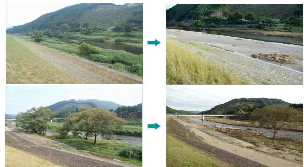
Photo 10 Fallen and discharged trees at upstream river channel before and after flood (The Japan Water Agency).
