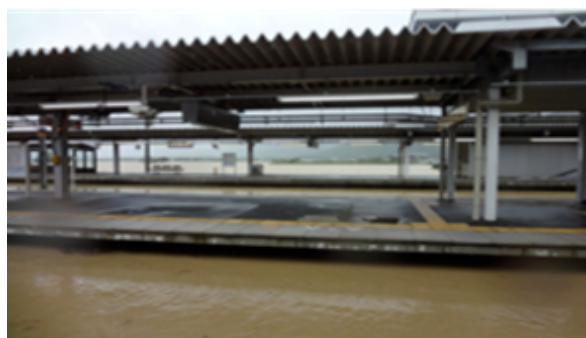
Photo 8 Kameoka station flooded just under platform home (Photo: Prof. Tomoharu Hori).
