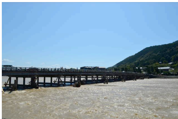
Photo 2 Togetsukyo Bridge looking from the upstream of the left bank of the Katsura river. Driftwoods reached the height of the bridge girder.
