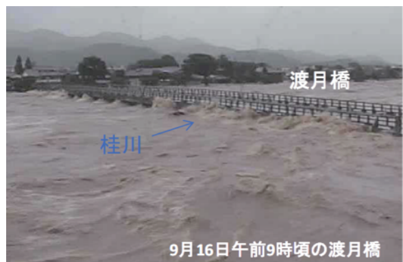
Photo 4 Flood water hitting Togetsukyo bridge around 9:00 on Sep.16
