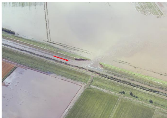
Photo 1 Damage in the Kenufuchi River, Hokkaido, Japan (Source: PWRI, Hokkaido)
