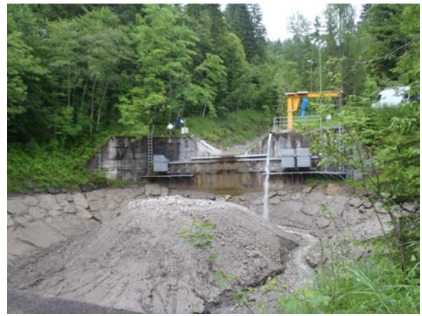
Photo 1 Observation site at Erlenbach and the retention basin
