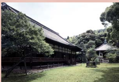
Shinden Hall, the Temple’s largest structure, features a hipped and gabled roof with tiles of wavy sections. The spirit of successive chief priests and related emperors are enshrined in the hall with the display of memorial tablets devoted to them.
