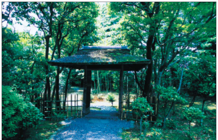
On the other side of the gate is a garden with large lawn areas. The aging structures are carefully maintained.
