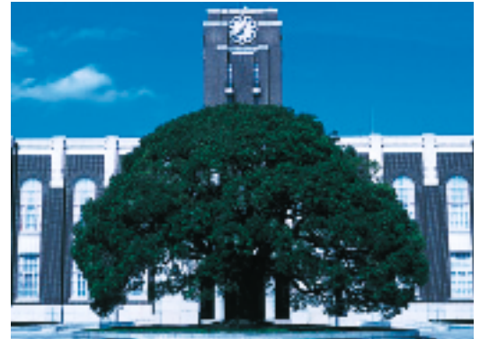
The Clock Tower, a symbol of Kyoto University, was renovated.
