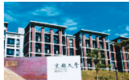
Sitting high on the hill, the General Research Buildings at Cluster A symbolize the Katsura Campus.
