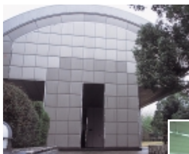
The FIFC is located about 2 km from the university in a quiet residential neighborhood, on a site facing the Takano River. The building has a marvellous atmosphere.
