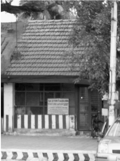
Photo 1. Façade of a Dikshitar's House
