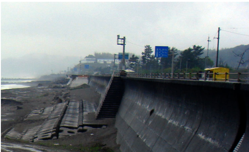
Fig. 3. Photo of seawall at a coast of Kochi, Japan.
