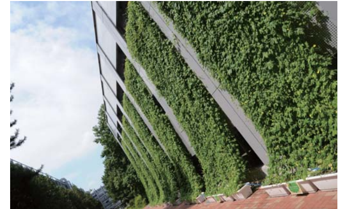
A “green wall,” which contributes to the reduction of building temperature and energy conservation
