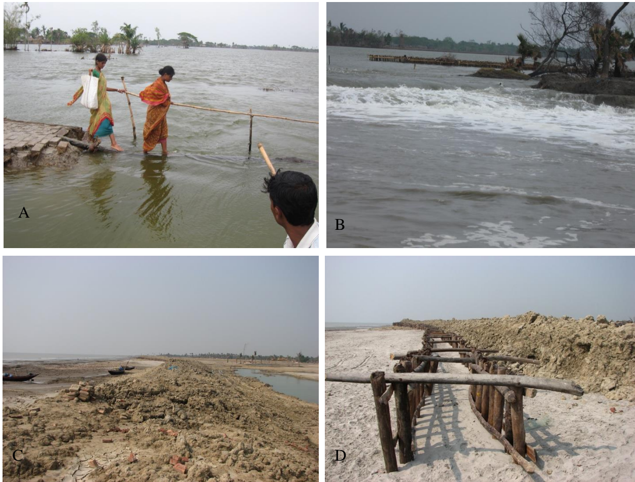
Figure 7.2. (A) Women crossing a breached embankment during Cyclone Aila (B) Overtopping of an embankment during Cyclone Aila (C) Sea dykes completely washed away in Cyclone Aila in Sagar Islands (D) New construction of embankments in Sagar Islands
