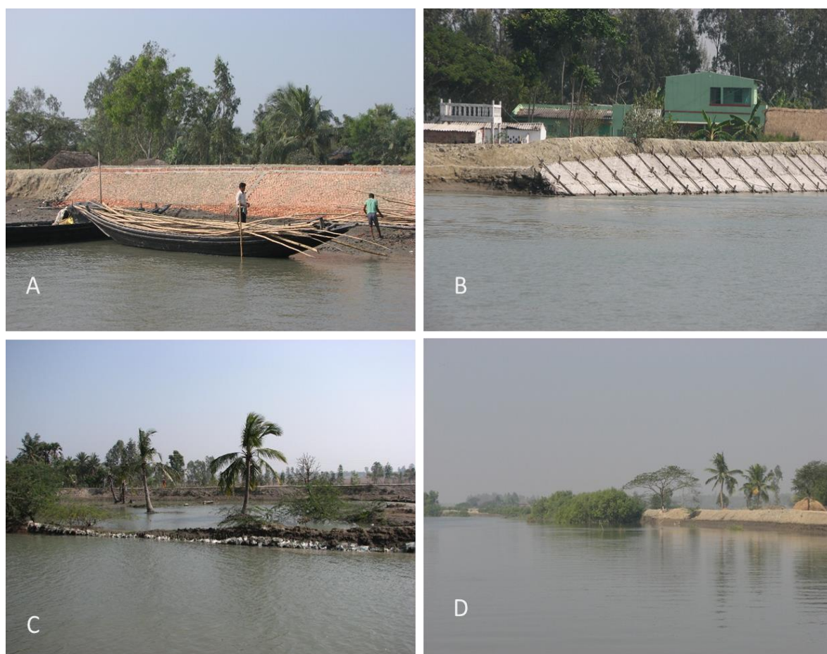
Figure 7.4. (A) Brick Lining of embankments in order to control erosion (B) Bamboo thatching to protect embankments (C) Damaged embankments and newly constructed embankments (D) Newly Constructed Earthen embankment in no protective lining.
