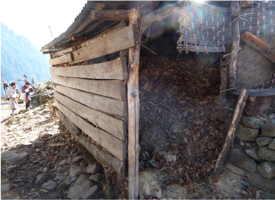
Figure 6.5 Storage shed for collected leaf litter in Gasa. January 2014
