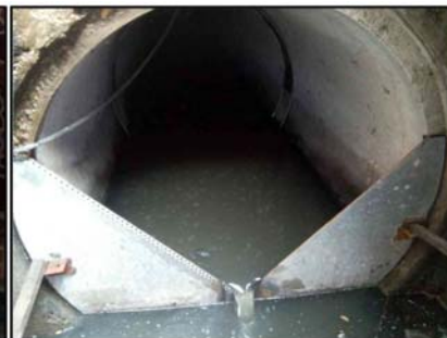
Figure 4-3 Installation of the weir into sewer pipe for flow rate measurement
