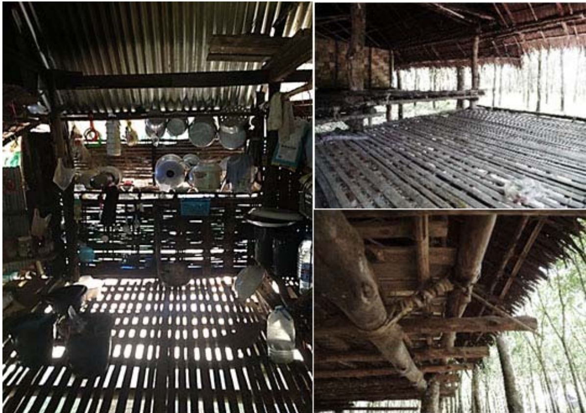
Figure 3.3 Kitchen area with shelf and bamboo floor (left), Bamboo floor steps (right-top) and joint details (right-bottom)
