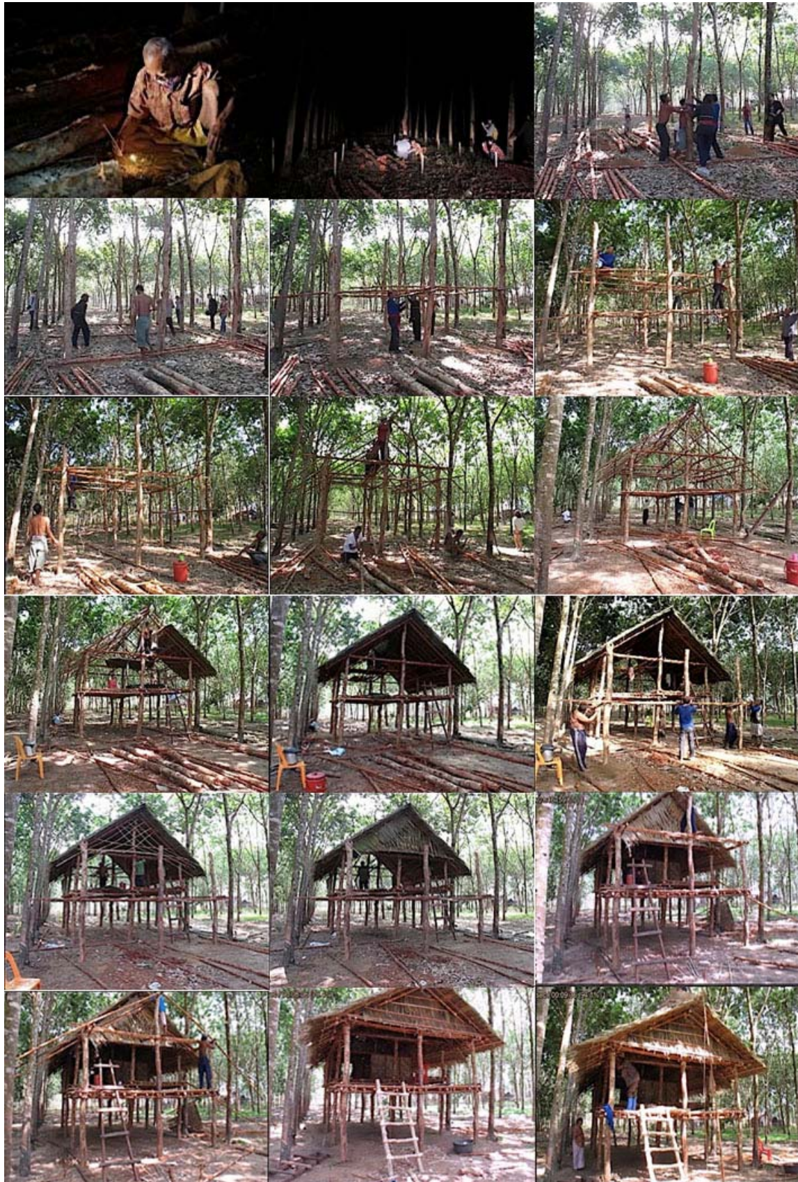
Figure 3.8 Construction process of the Moklen ethnic house
