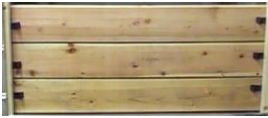
Photo 2 flood board ( wood board )
