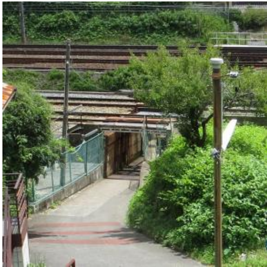
Photo 1 Underpass (passageway under railroad)
