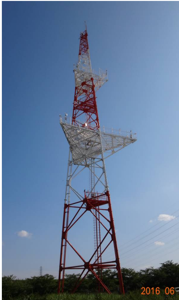
Photo 1 55-m tall meteorological tower at Ujigawa Open Laboratory
