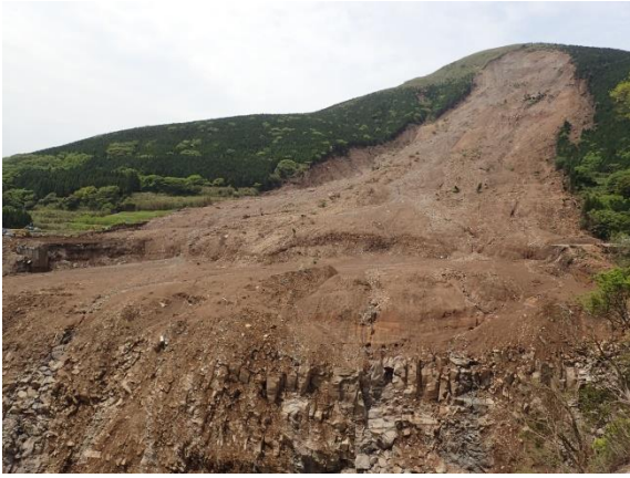
Fig. 29 The landslide near Aso-Ohashi
