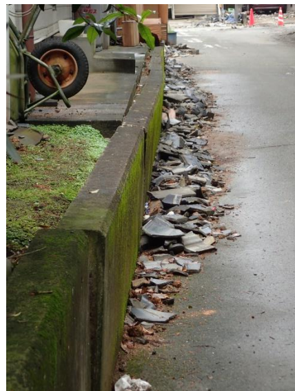
Fig. 14 The inclined concrete retaining wall
