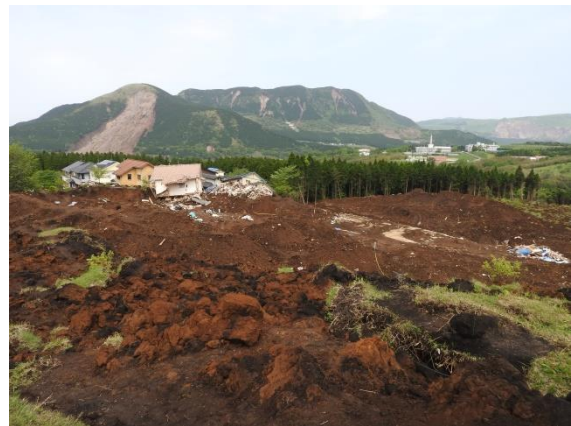
Fig. 32 600m away to the downstream involving the great damage of the houses
