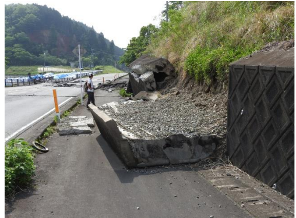
Fig. 27 a fallen retaining wall on the fault
