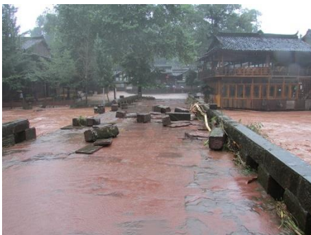
(e) Destroyed bridge on spot (e)
