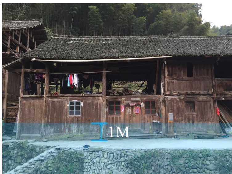
Figure 4. 10 A building without flood countermeasures was inundated up to about one meter
