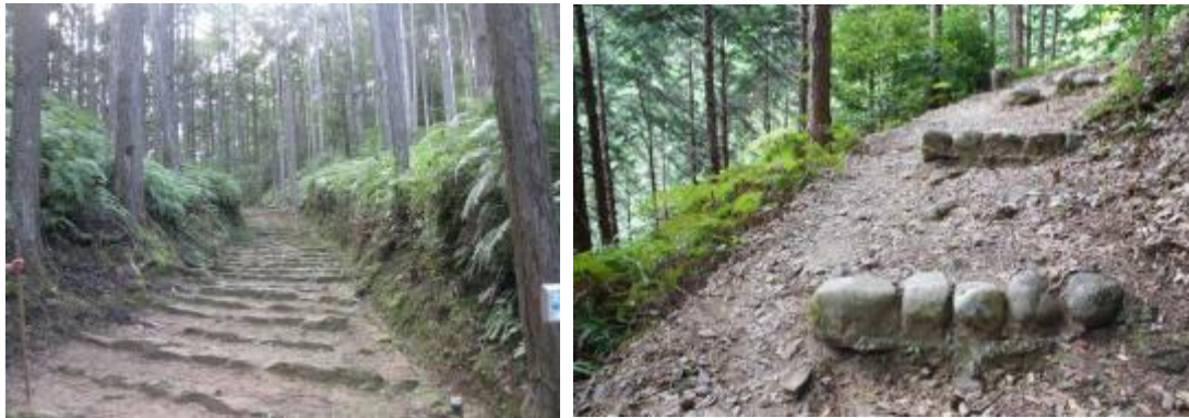
Figure 4.5 Stone steps along the Nakahechi Route. a. left Steps that are thought to date back to the Edo era. The native rocks are arranged according to the adjacent landform and trail widths, allowing the natural flow of water drainage on the side; b. right Steps constructed during the restoration project 1978–1982. The stone structures fixed by concrete at the bottom are determined with a fixed length, accelerating water flow through the surface. A second tread is also shown in the photo, indicating that a severe incision at the bottom of the stone structure caused difficulties for walking.
