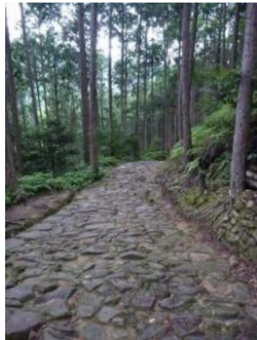
Figure 4.1 Stone pavements that can be observed along the Nakahechi Route, estimated to have been constructed during the Edo era.
