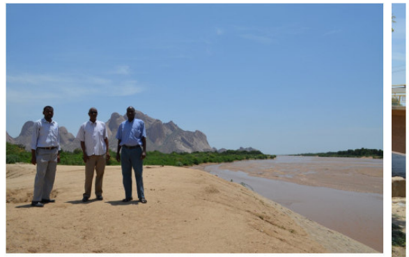
Plate 9: View of the Gash Protection embankment
