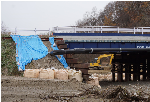
(a) Kiyomi Bridge over Tokoro River
