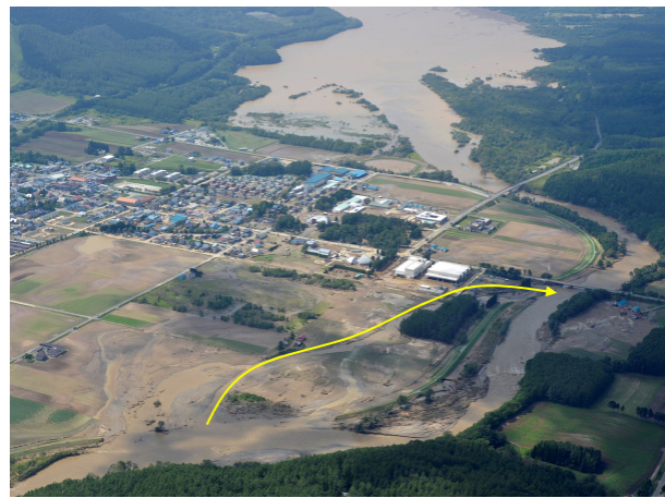
Fig. 11 Inundation and return flow around Sorachi River (photo by Pasco Co.Ltd.)
