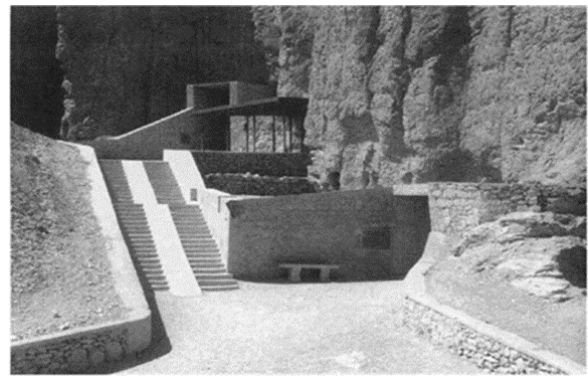
Fig. 4 The protective wall
