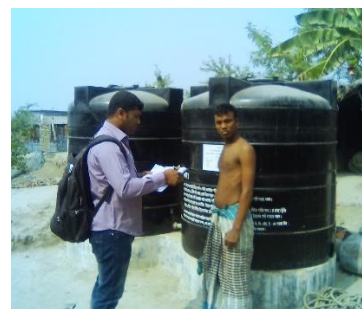
(c) Waters tanks of a home based Rain Water harvesting System
