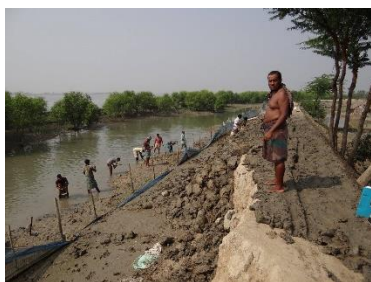
(a) Repair of embankment
