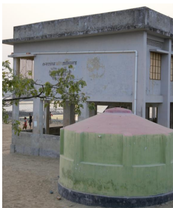
Photo 3 A rainwater harvesting system installed at a school
