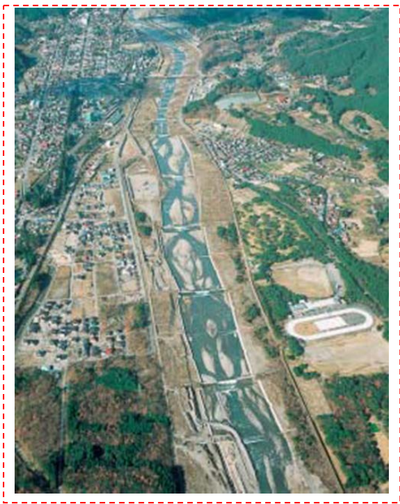
Fig. 14 Japanese river with structural measure Source: arranged from Sabo in Japan (MLIT)
