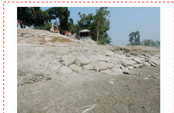
Fig. 4 Sandbags on the embankment for preventing erosion (Fulcchari, Gaibandha in Dec. 2014)
