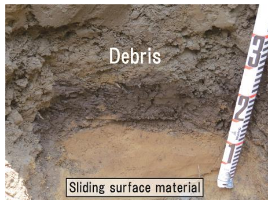
Fig. 11 A sliding surface formed in the upper portion of the Br layer with lava block in KGC-1.
