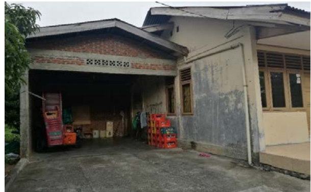
Figure 4.19 Storage area (extension)
