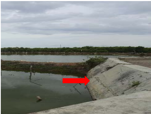
Figure 4.38 Poorly built seawall as of 2016
