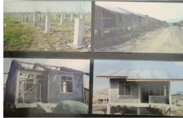
Figure 5.22 Housing reconstruction (Source: Gampong Lambung Office)
