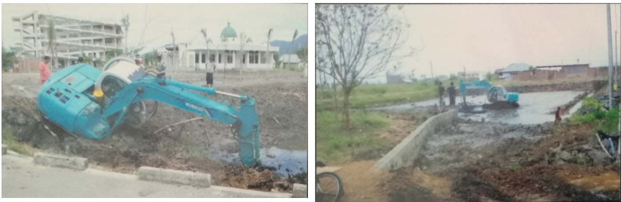
Figure 5.33 The process of making kolam ikan (fishpond) (Source: Gampong Lambung Office)
