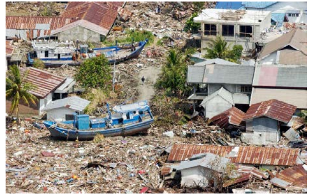
Figure 1.3 Massive destruction in Banda Aceh after the 2004 Indian Ocean Tsunami Disaster (Source: The United Nations, 2004)
