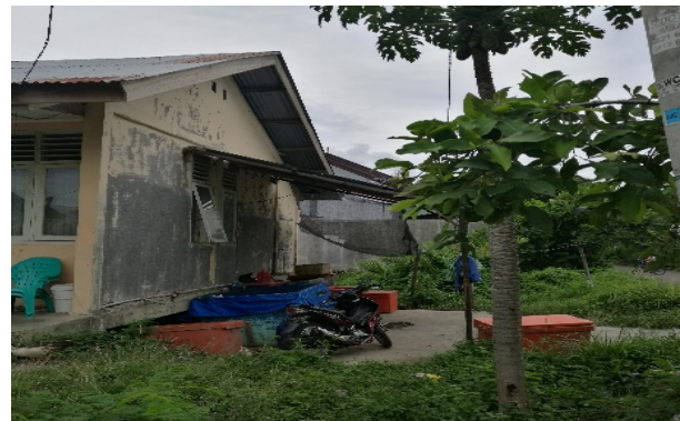
Figure 5.24 Roof extension was made for livelihood equipment storage
