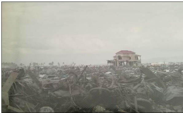
Figure 5.9 The only house remaining after the tsunami (Source: Gampong Lambung Office)
