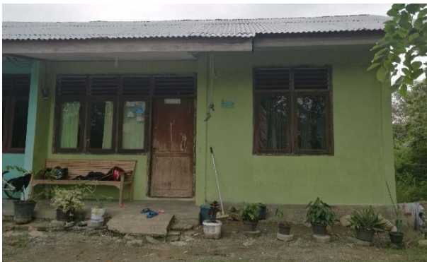
Figure 5.19 House constructed by World Vision
