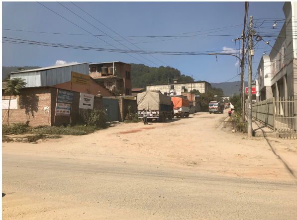
Internal road in Balaju Industrial District
