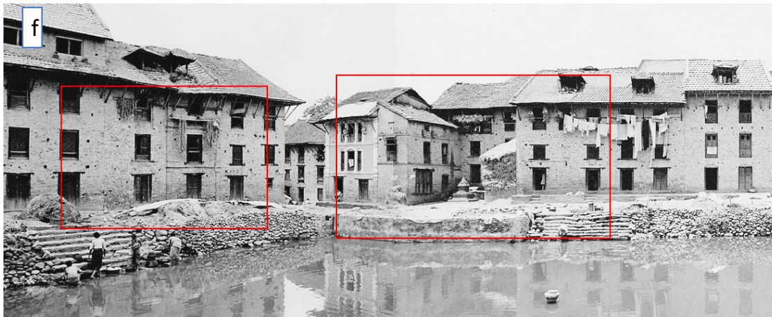
Figure 6.20 f. Photograph of the row houses near De-pukhu taken in 1968 with symmetrical openings and buildings made of brick in mud mortar with tiled roof. (Source: Thomson et al., 1968)
