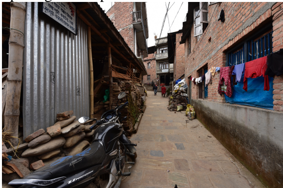
Shop operating from temporary shelter
