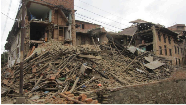
Building collapse near De-pukhu
