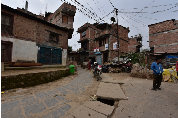
Photographs showing change in door openings in shop
