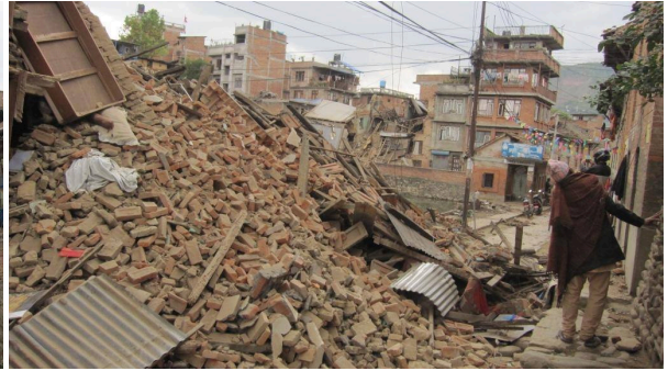
Blocking of road due to collapsed building
