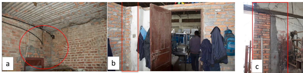
Figure 5.9 (a, b, c) Repair works observed in the BID
