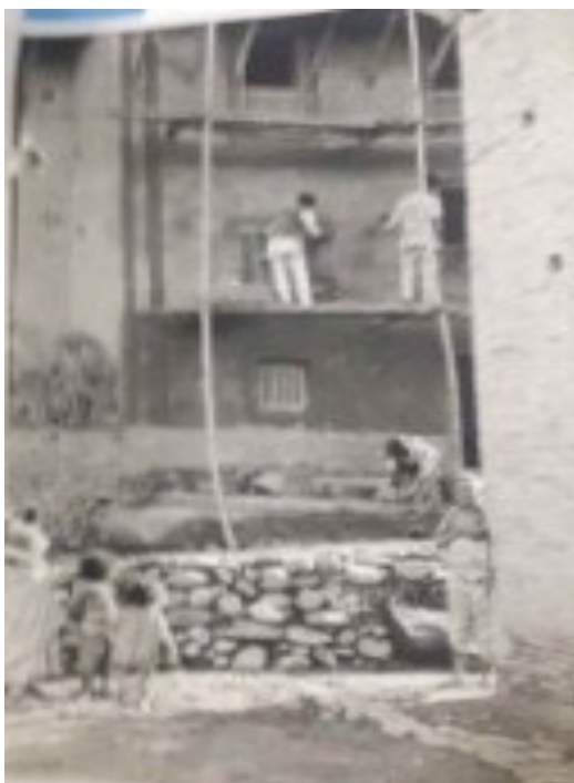
Construction/repairing work in Bungamati
