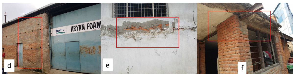
Figure 5.9 (d, e, f) Repair works observed in PIE
