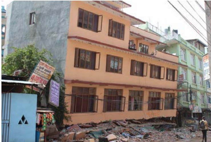
Figure 3.2 Damages to buildings in Balaju Area
