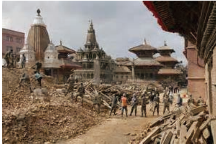
Figure 3.3 Damages to Patan Durbar Square near to Patan Industrial Estate
